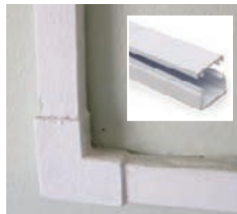
Two pieces to handle, awkward to install, lids can detach to create on-going maintenance demands.
