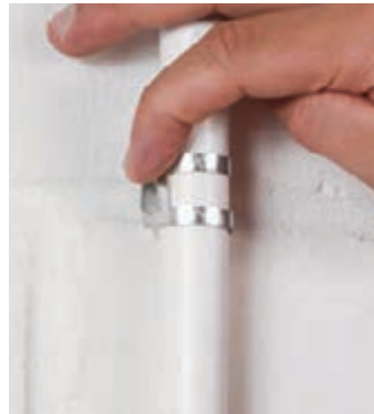
Secure conduit with locking tab
