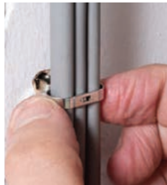
Insert cable(s) before squeezing the smooth head
